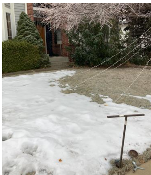
Figure 4. A curb stop used to return water service to a standing structure for flushing and sampling
