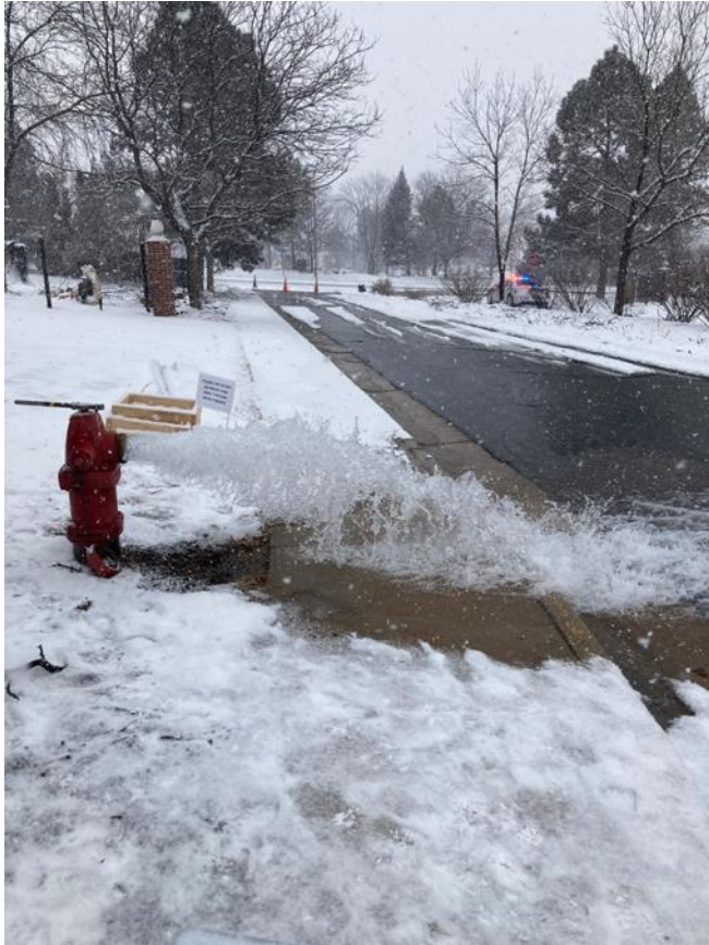
Figure 2. A hydrant being used to flush water in the fire impacted area
