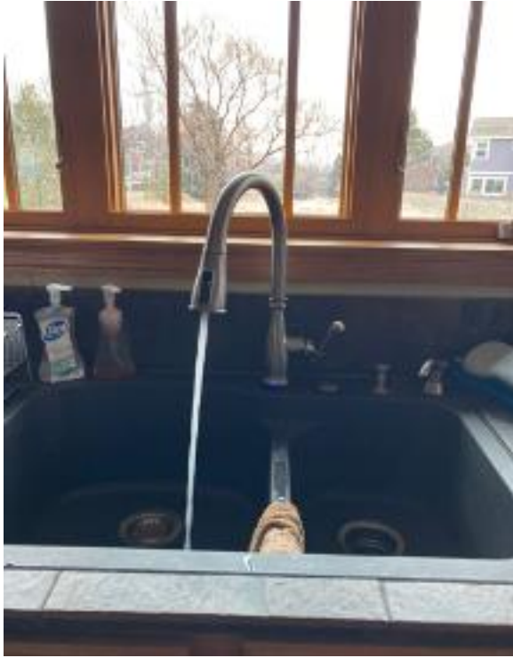
Figure 5. A sink being flushed during sample collection
